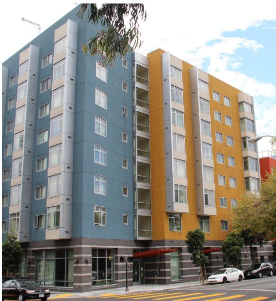
Parcel C. 701 Golden Gate Ave Street
